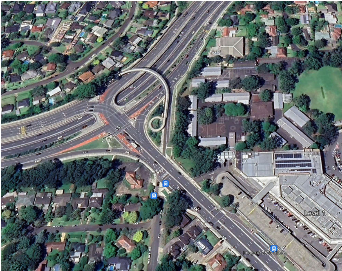
Figure 3.6 – Photo showing new intersection with Warringah Road and Forest Way
